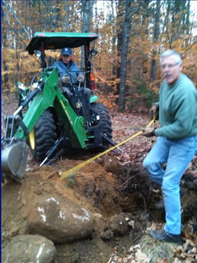
Erosion control work, Page Hill Trail, October 2010
